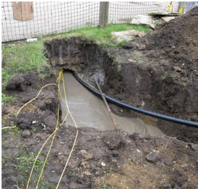
Tracer wires being pulled through the borehole along with the pipe.
