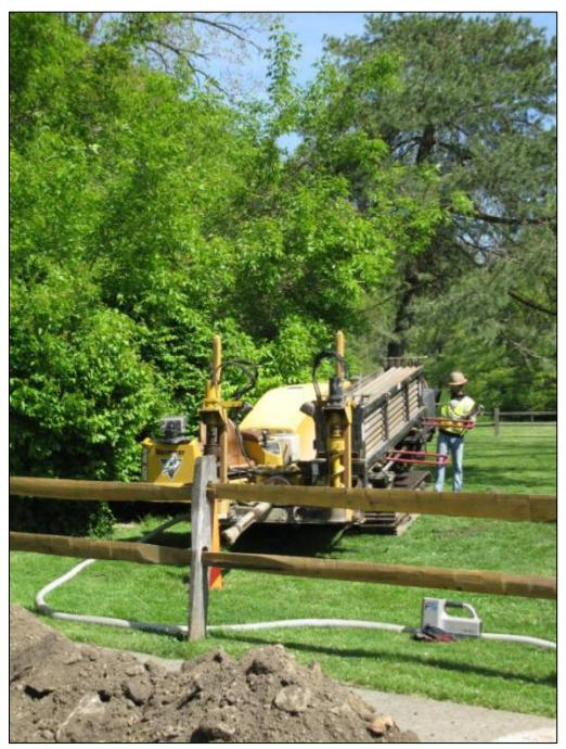
Figure 50. Vermeer HDD Machine at the Job Site
