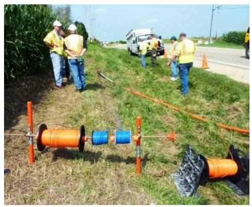
Figure 43. Four tracer wires used during HDD pipe installation
