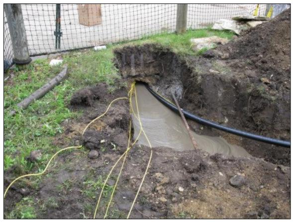
Figure 57. Tracer Wires being Pulled through the Borehole along with the Pipe
