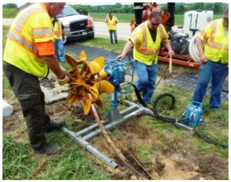
Figure 49. Three Tracer Wires being Pulled out of the Ground
