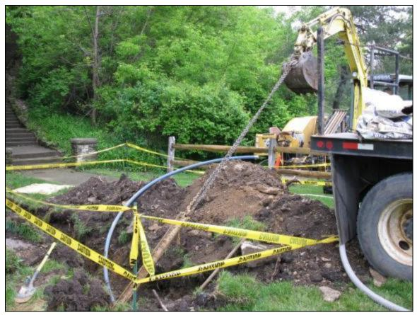
Figure 58. Pipe and Wires being Pulled out by Backhoe
