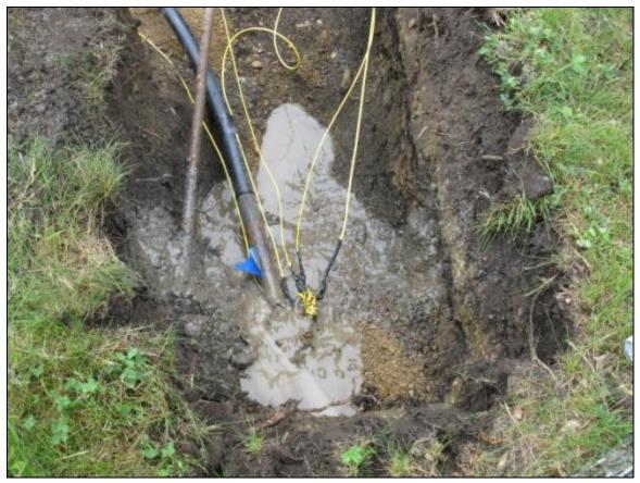
Figure 56. Five Tracer Wires Used during HDD Pipe Installation
