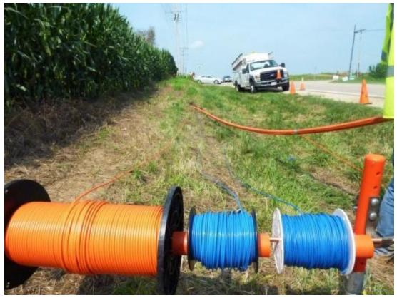
Figure 45. Tracer Wires during Pull In
