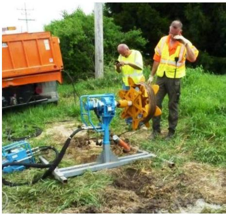
Figure 48. Three Tracer Wires being Pulled out of the Ground
