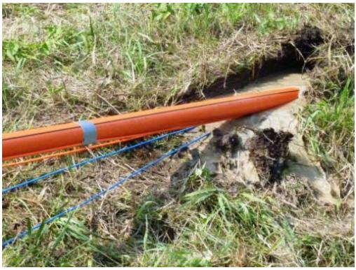
Figure 44. Tracer Wires being Pulled in with Pipe
