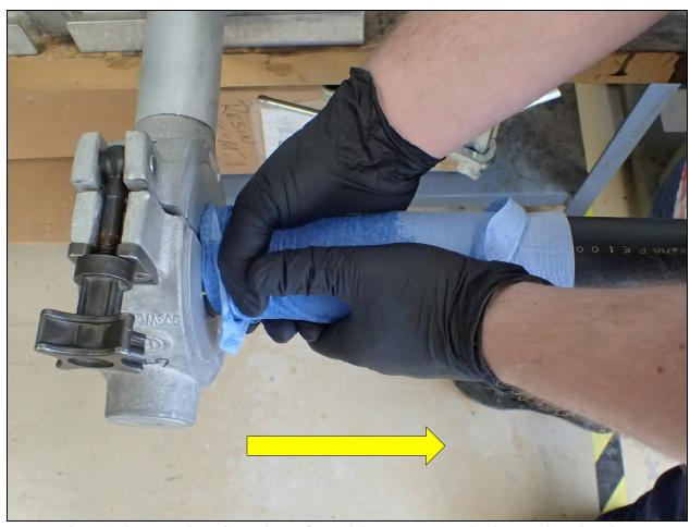
Figure 160. Wrapping of the pipe before wiping pass, arrow indicates wipe direction
